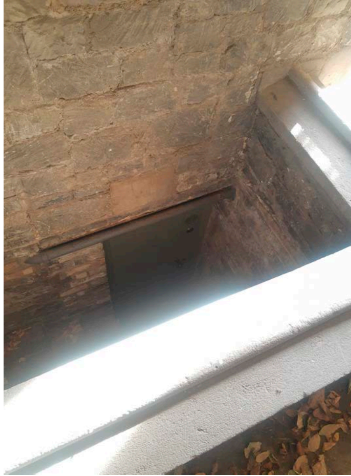
Figure 13: Cottage plant room door, located at the bottom of a staircase.
