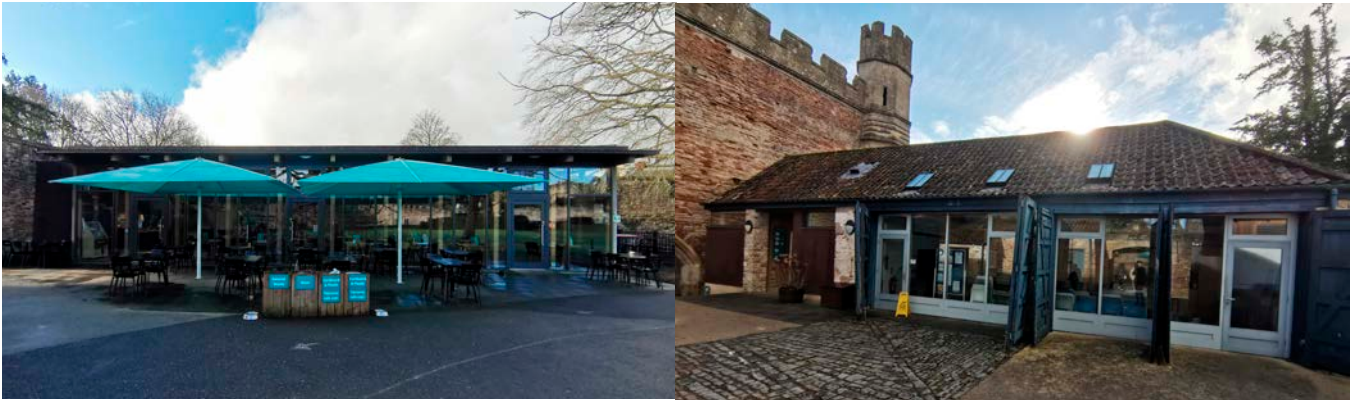
Figure 9: The cafe (left) and learning centre and toilet block (right), heated by the WSHP.
