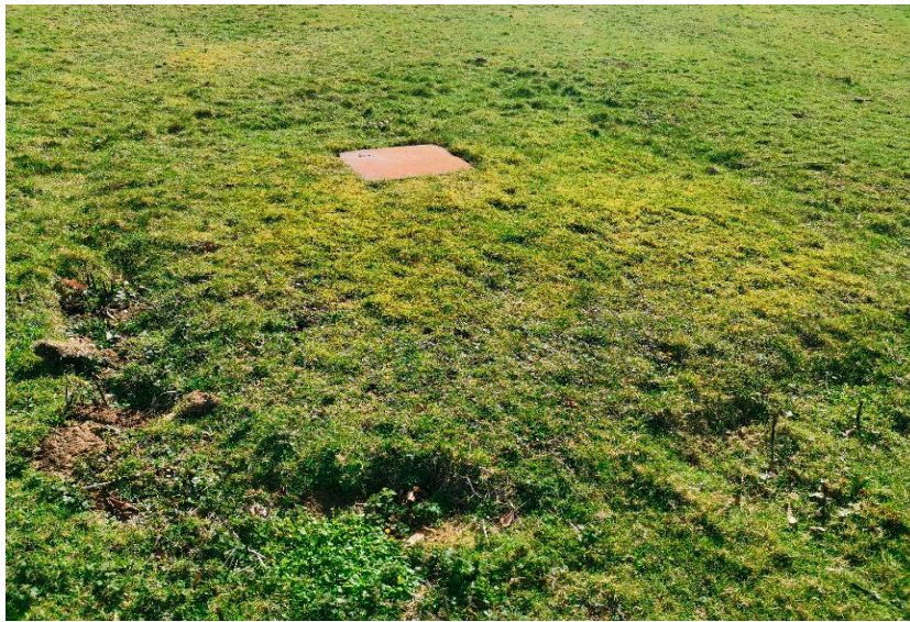
Figure 24: The raised ground around the manifold collector chamber.
