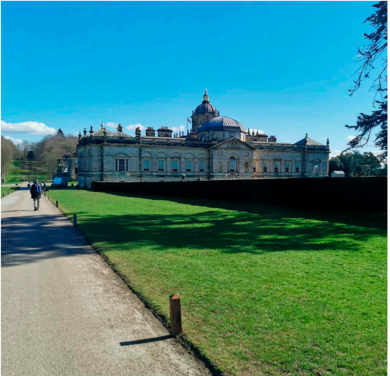
Figure 20: Site 4, North Yorkshire.
