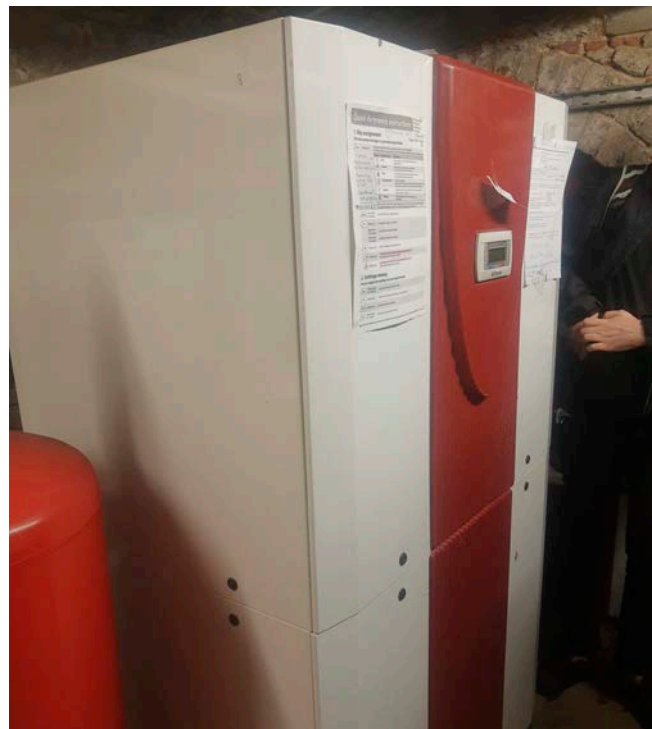
Right: Figure 32: The Dimplex GSHP in the basement plant room at Site 5.
