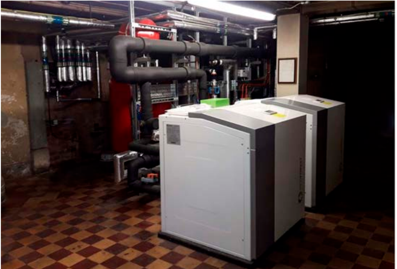
Figure 13: GSHPs in the basement plant room.
