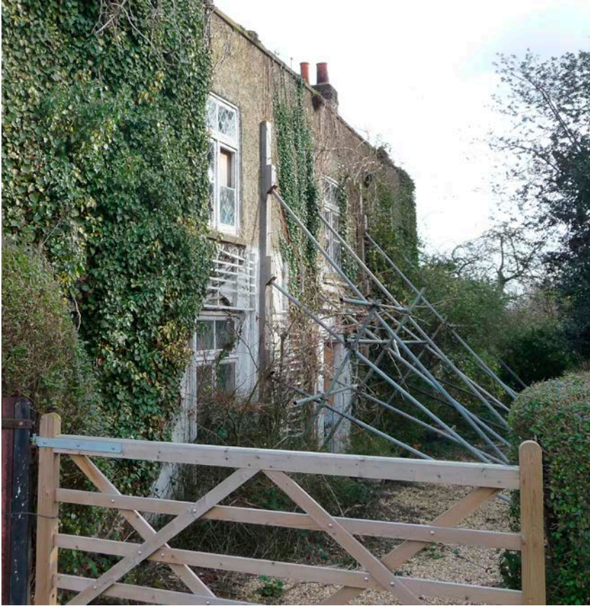
Figure 8: Steel scaffold shoring. Crossways. Again these shores generally have out of plane bracing for stability.
