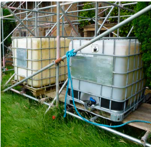
Figure 44: Precast kentledge to resist uplift. © Benchmark Scaffolding
