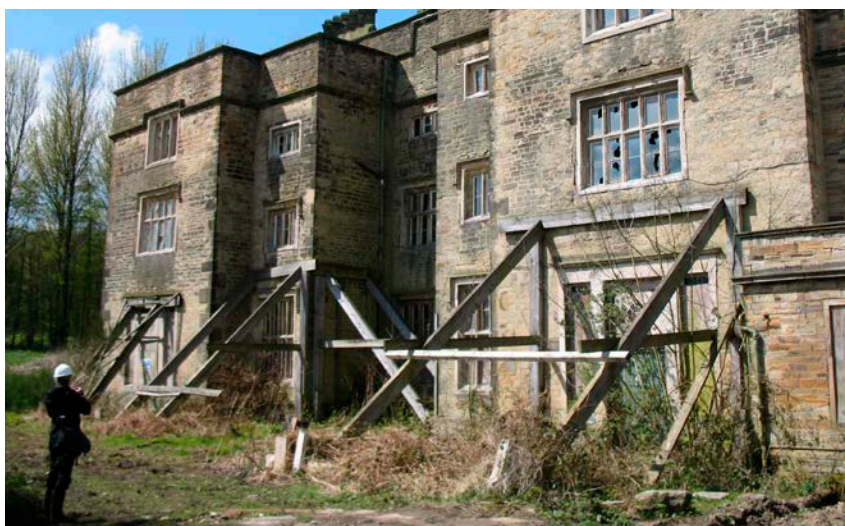
Figure 7: Timber shoring. Winstanley Hall. Note these shores generally have out-of-plane bracing for stability.
