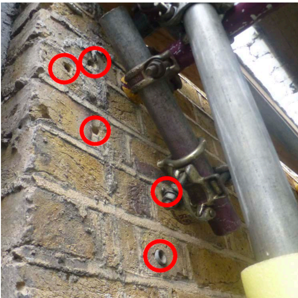
Figure 5: Drilled anchor tie and holes in masonry from previous scaffold interventions.
