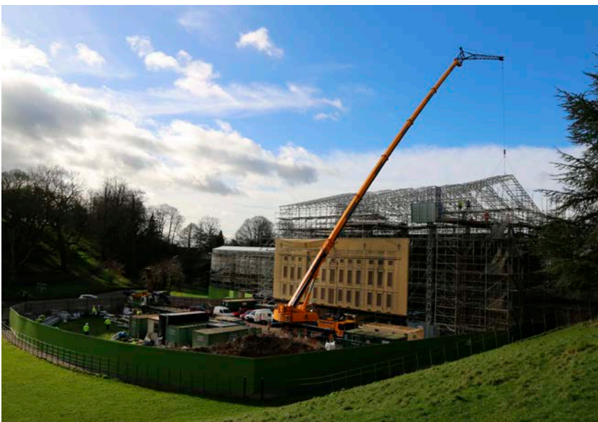
Figure 58: Crane lifting temporary roof into place.
