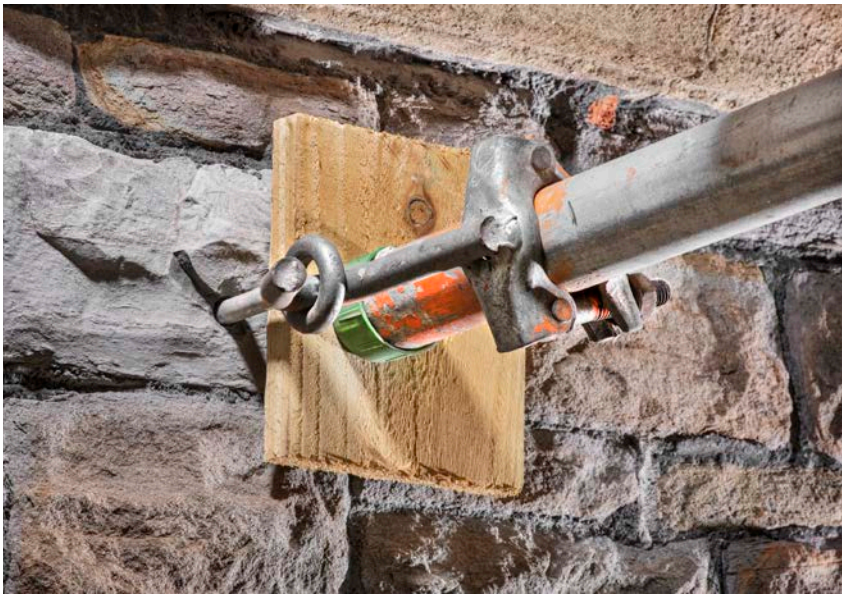
Figure 43: Scaffold ring bolt in a drilled resin anchor socket. © Historic England Archive
