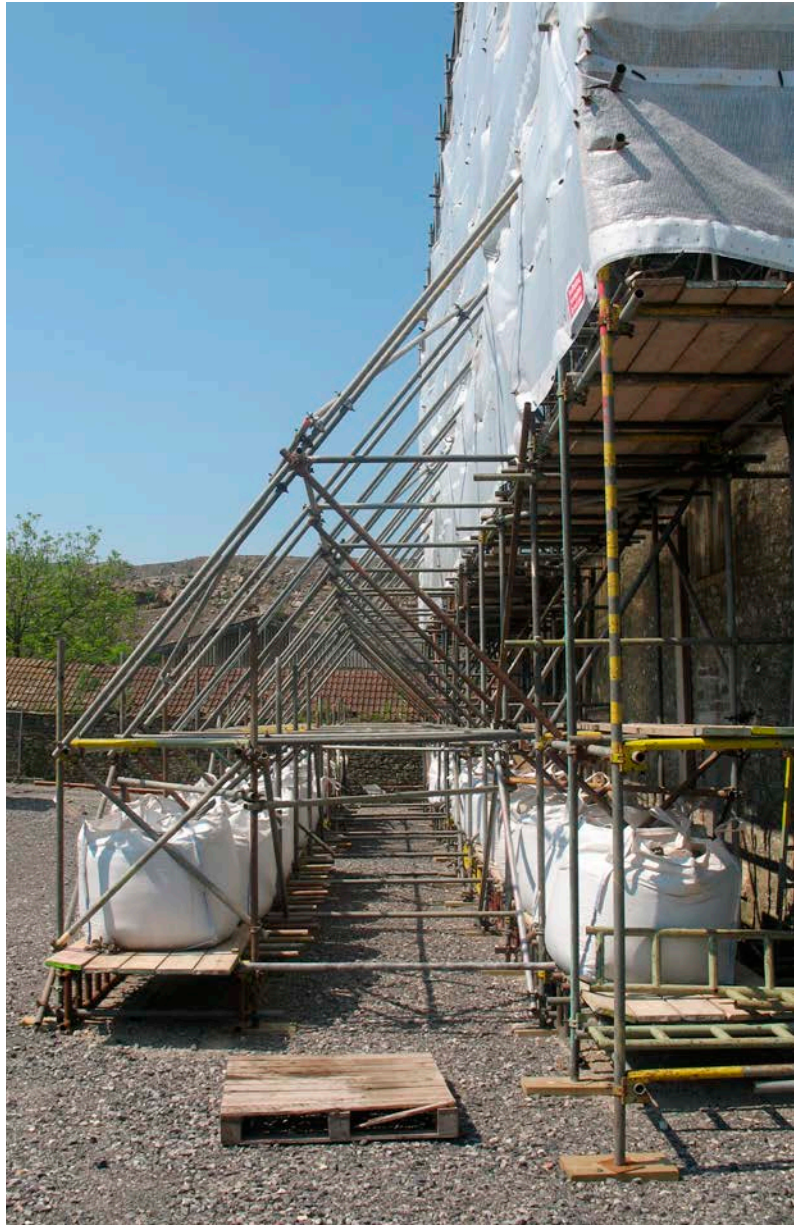
Figure 44: Precast kentledge to resist uplift. © Benchmark Scaffolding
