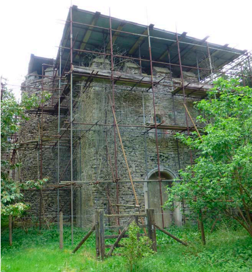
Figure 51: Corroding free standing scaffold.
