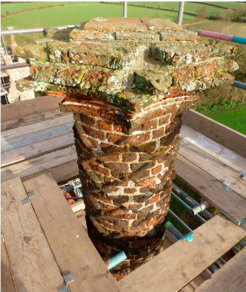
Figure 3: Scaffold around a chimney but not in contact. Ideally the gap should be protected.
