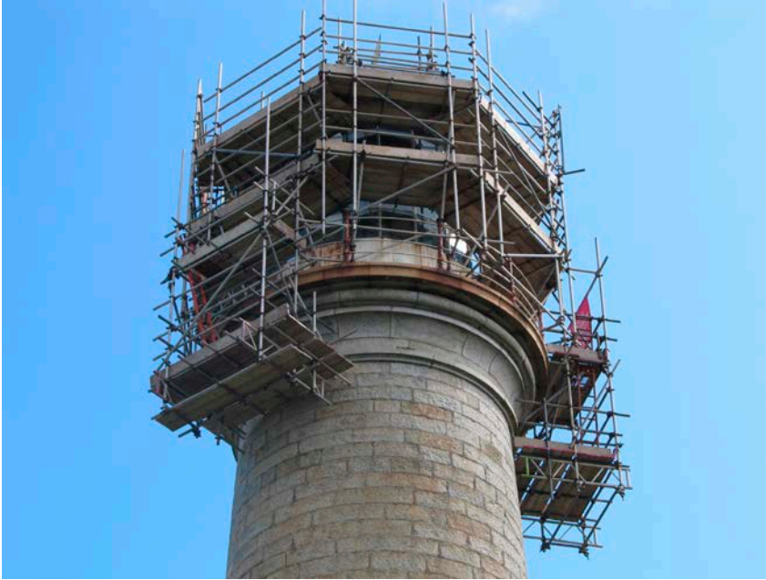
Figure 15: Slung scaffold used for repairs to a tall chimney.
