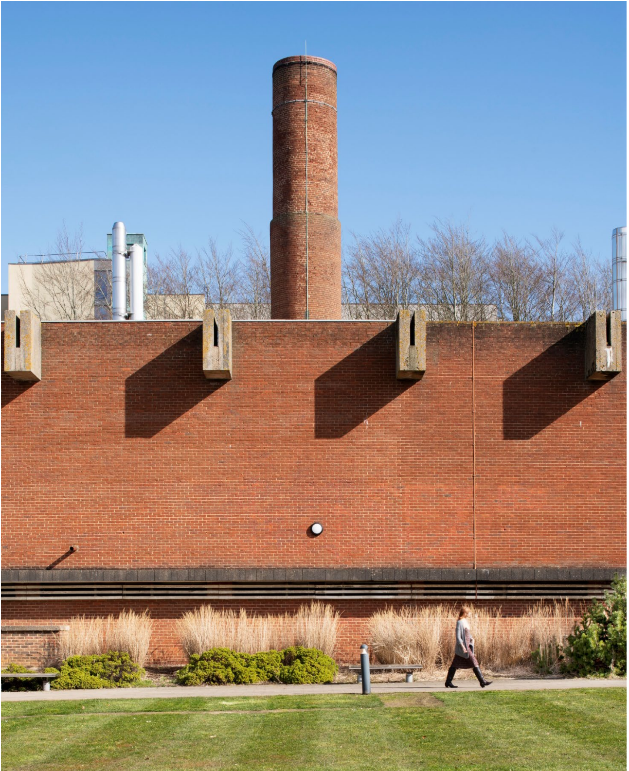
Boiler House designed by Sir Basil Spence, University of Sussex, Brighton, East Sussex. Included on Brighton and Hove's Local Heritage List. James O. Davies © Historic England Archive DP439657
