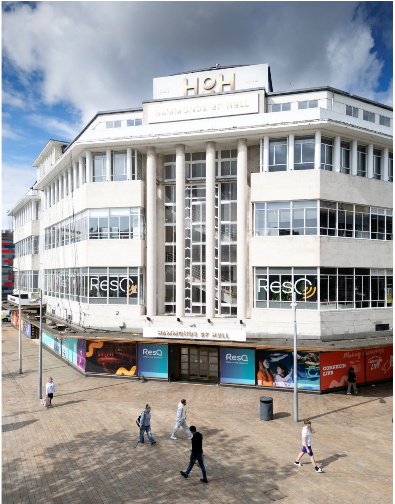
Hammonds of Hull (later House of Fraser), Ferensway, Kingston upon Hull. Included on Hull's Local Heritage List. Alun Bull © Historic England Archive DP486117
