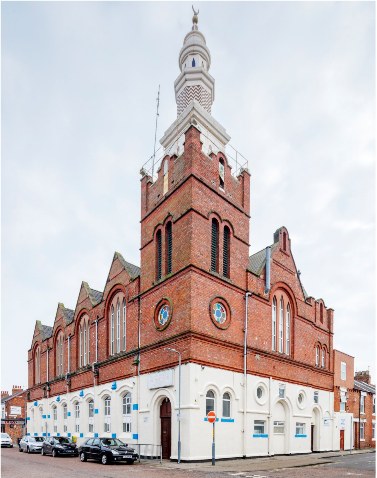
Jamia Masjid Al-Madina, Waterloo Road, Middlesbrough, Tees Valley. Included on Middlesbrough's Local Heritage List. Alan Bull © Historic England Archive DP486736
