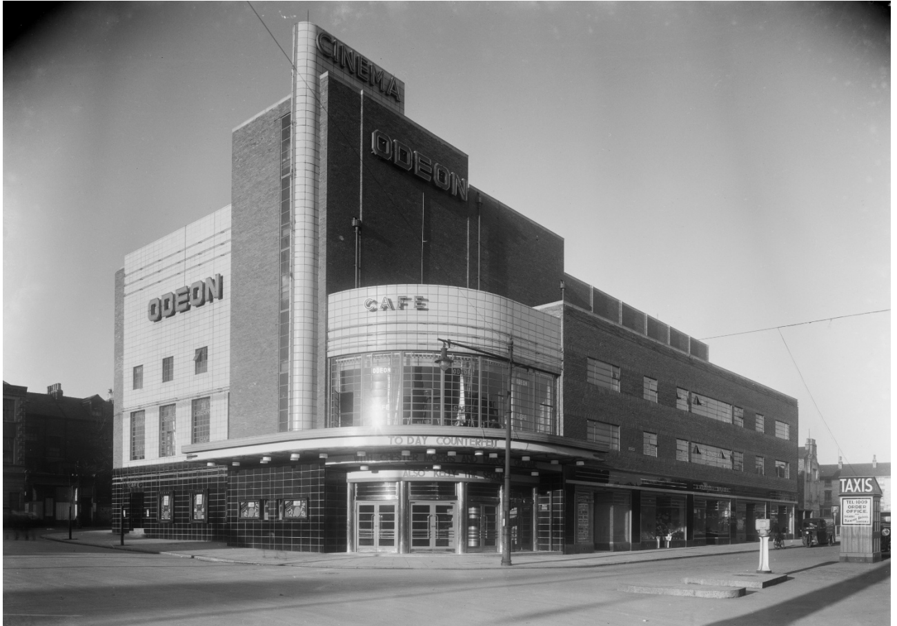
Figure 11 - The new Odeon style shown at Scarborough, North Yorkshire, opened in 1936. Photographed 1936. Listed, Grade II, 1243674 [John Maltby © Historic England Archive BB87/03389]
