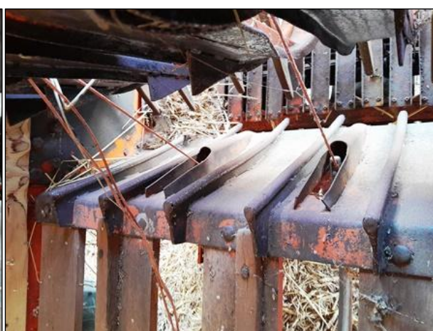
Steel bars on rib leading edges but overall height too low - (Could be Better)
