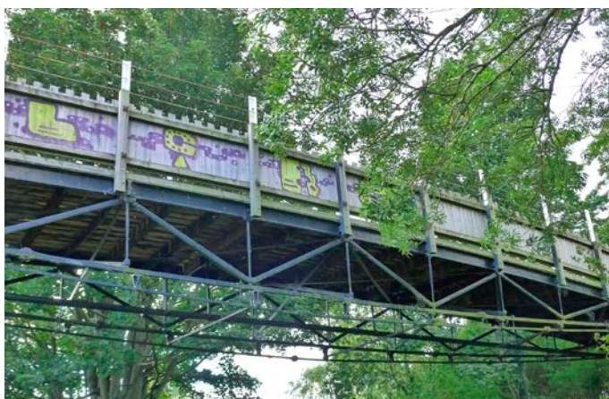
Figure 8 (above): The western elevation of the lenticular truss bridge, DAE2/12. © Mr Brian Wilcockson (Source: Historic England Archive IOE01_01853_03)
