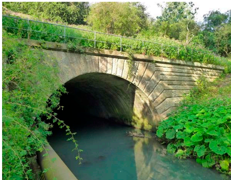
Figure 6 (above): The southern portal of culvert DAE2/8 taking the River Gaunless beneath the railway. © Historic England
