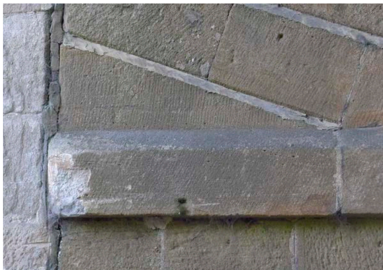
Figure 3 (above): Detail of the springing of the arch barrel of DAE2/4, showing the stones of the impost banding cut as one with the first course of stones in the arch barrel to help prevent the barrel sliding over the abutments. © Historic England
