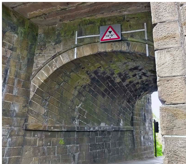
Figure 1 (left): The eastern elevation of railway underbridge DAE2/4, masked by later track widening. © Historic England
