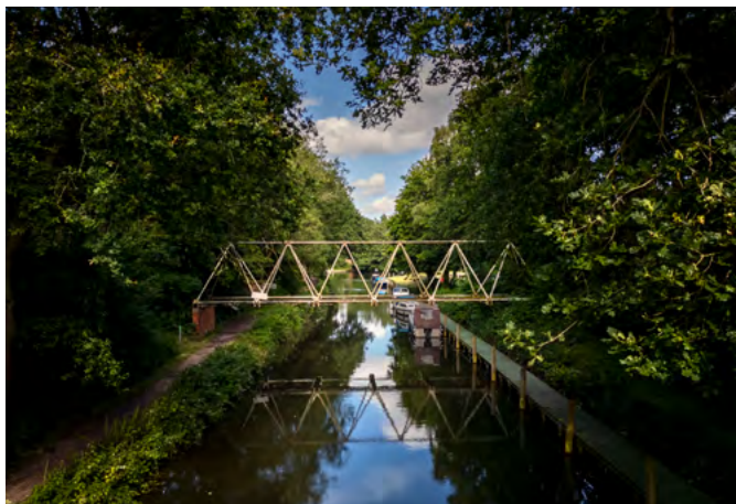
The Inglis Portable Military Bridge over the Basingstoke Canal, Aldershot, Hampshire. The component-based design allows a team of 12 soldiers to erect the structure in around 15 minutes.
