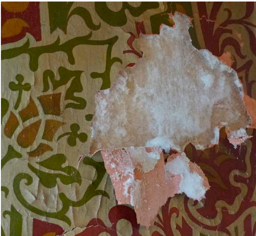
Figure 9: Delamination and flaking of paint layer caused by salt activity.
