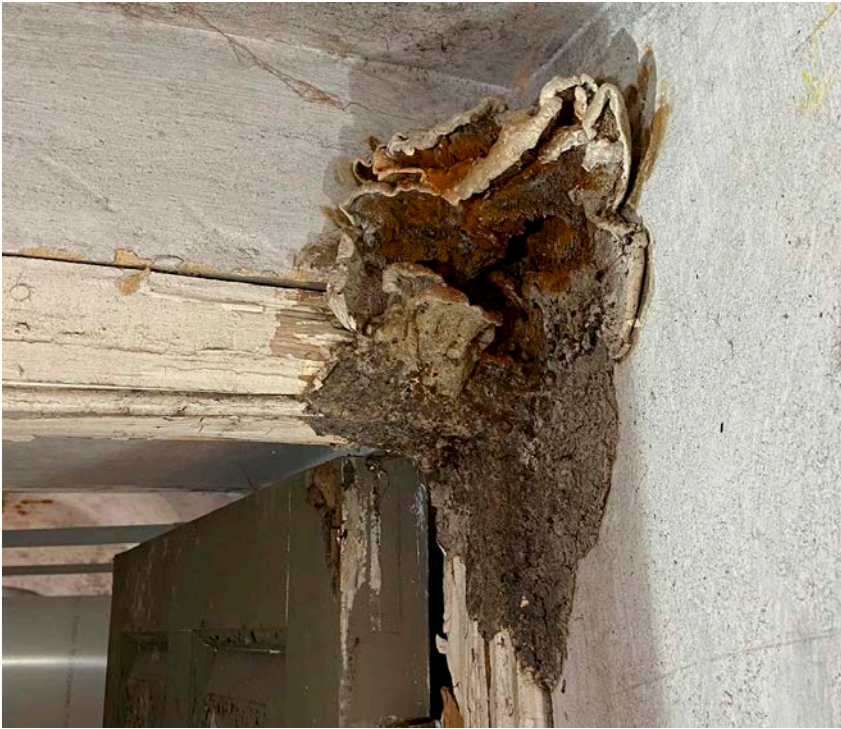
Figure 10: Dry rot caused by high moisture levels resulting from water ingress. © Tobit Curteis Associates
