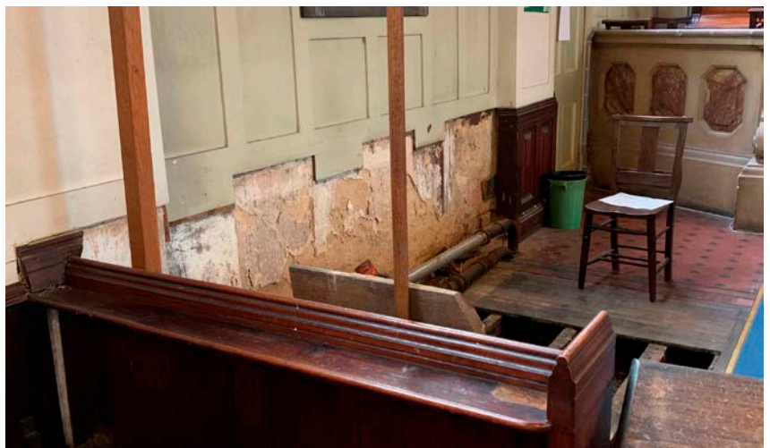
Figure 22: Damage to the base of the wall caused by a burst water pipe.
