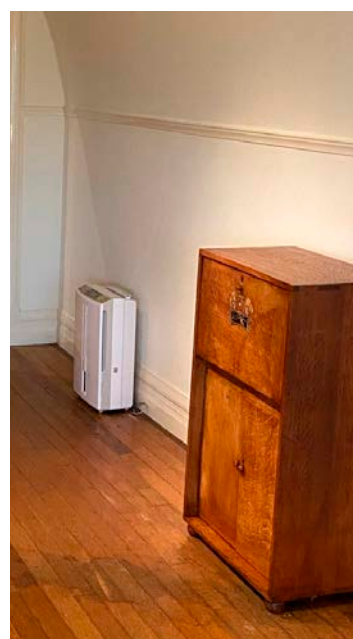
Figure 42: Mechanical units can have unexpected effects. Heat output from dehumidifiers may be beneficial, but can also cause damage if located next to a sensitive artefact or piece of furniture. Thermal image (left) shows the spread of the heat output from the dehumidifier in this example (right, room in normal light). © Tobit Curteis Associates
