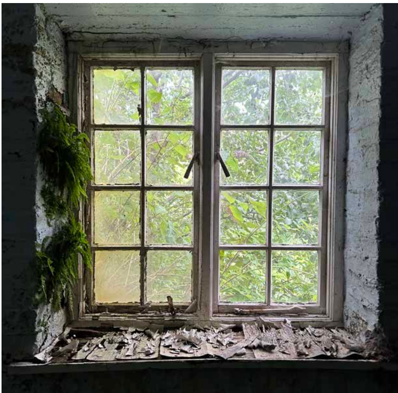
Figure 6: Condition of window pre-development, 2023. © JDDK Architects Ltd.
