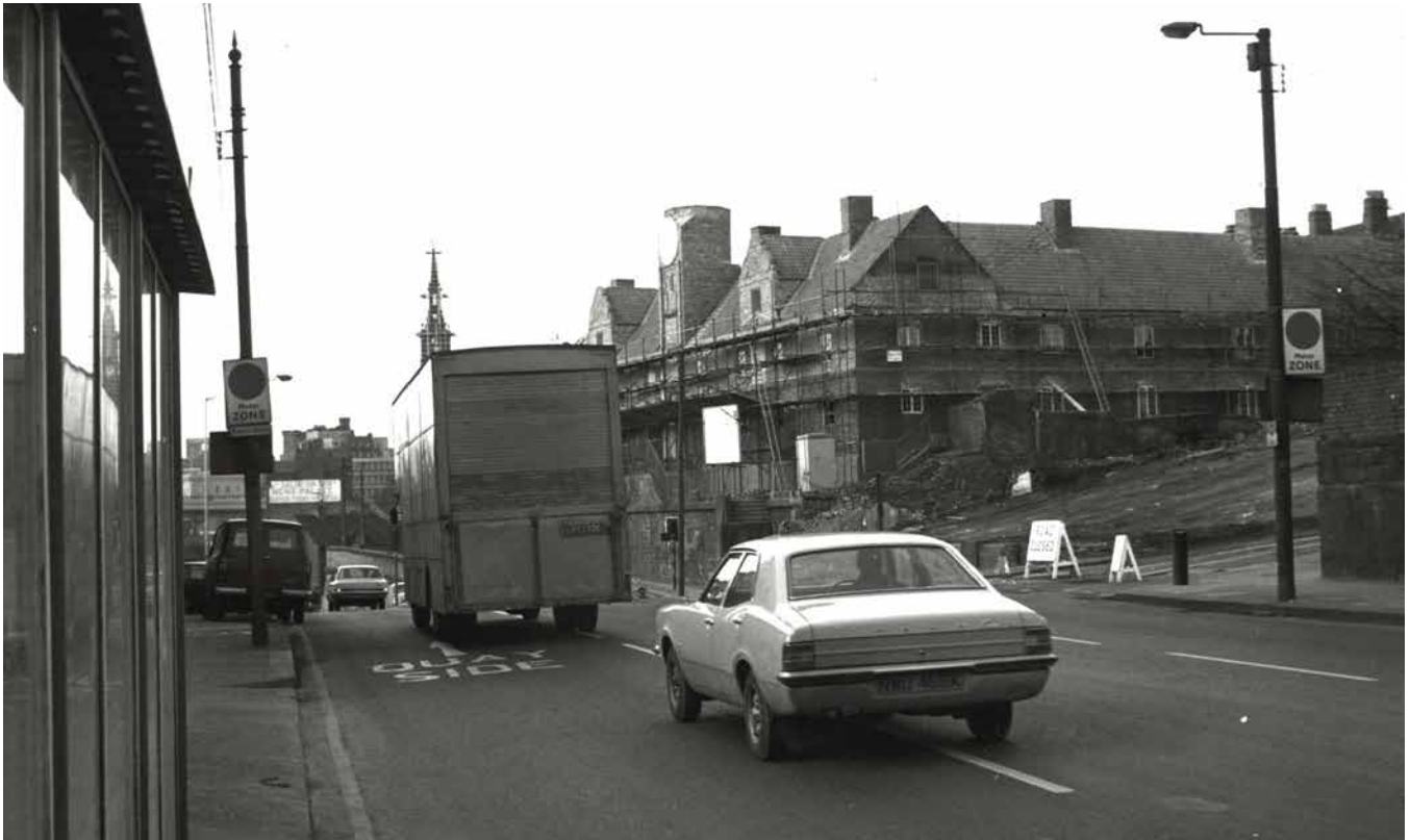
Figure 2: South-east and north-east elevations during building works, 1973. © Newcastle Libraries.
