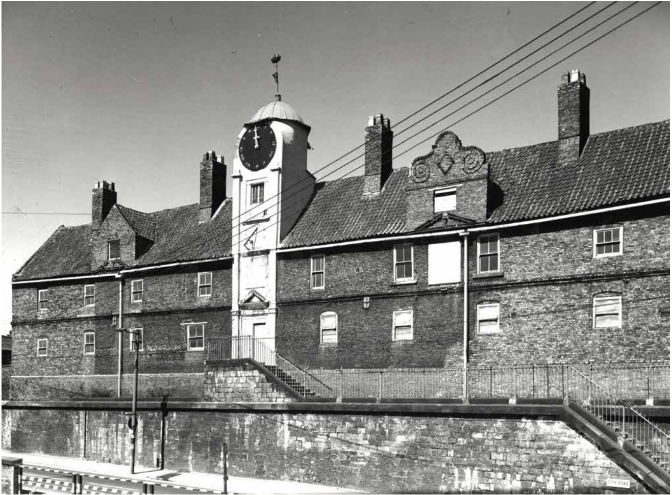
Figure 5: South-east elevation of Keelmen's Hospital, 1969 (pre-1973 works). © Newcastle Libraries.
