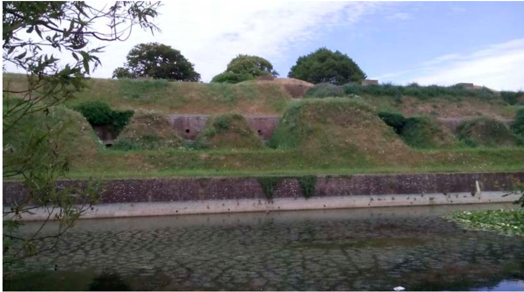
Figure D2: External view of the store.
