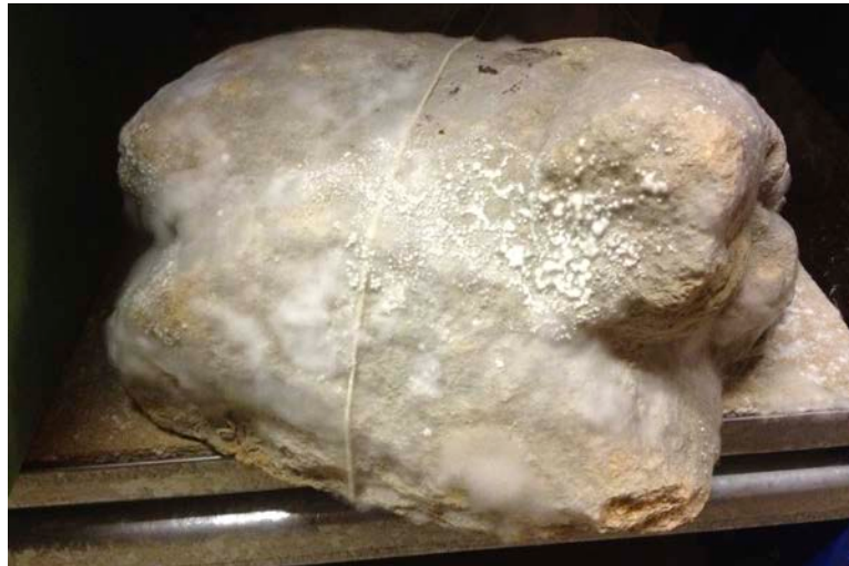
Figure D4: An example of the mould, which appeared as a white surface bloom on stonework, pallets and shelving in storage.
