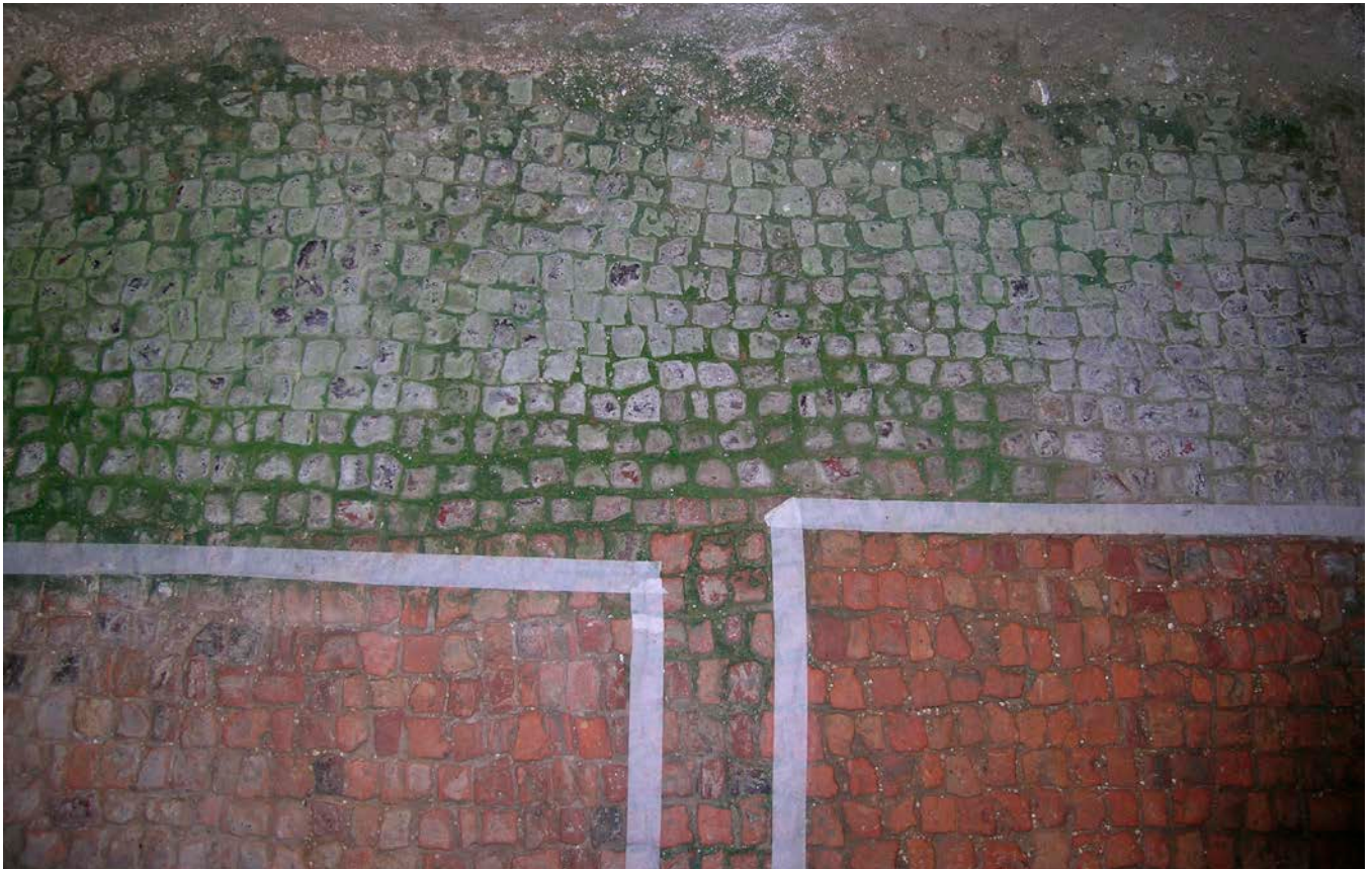
Figure C2: Trial area 1 (left) and trial area 2 (right), demarcated by tape, after UVC irradiation and wet cleaning.
