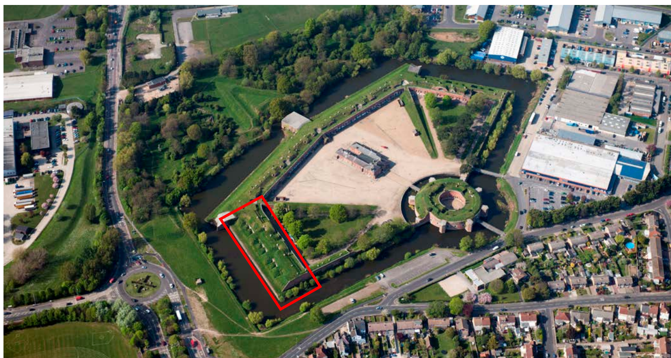
Figure D1: Fort Brockhurst from above, with the store in the bottom left area.
