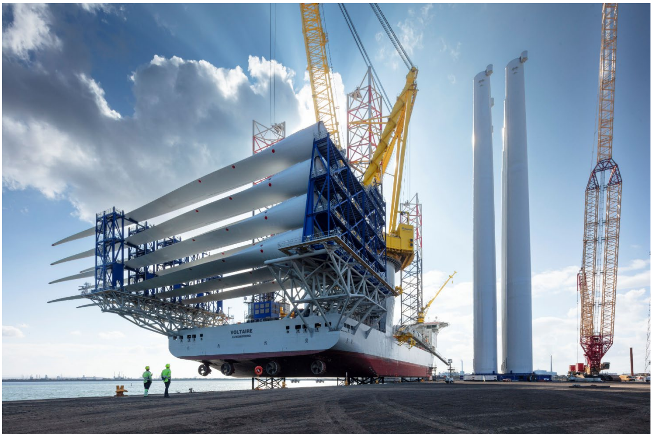
The installation yard for Dogger Bank A,B,C Wind Farm at Able Seaton Port, Hartlepool, County Durham. © Historic England Archive, DP486617.
