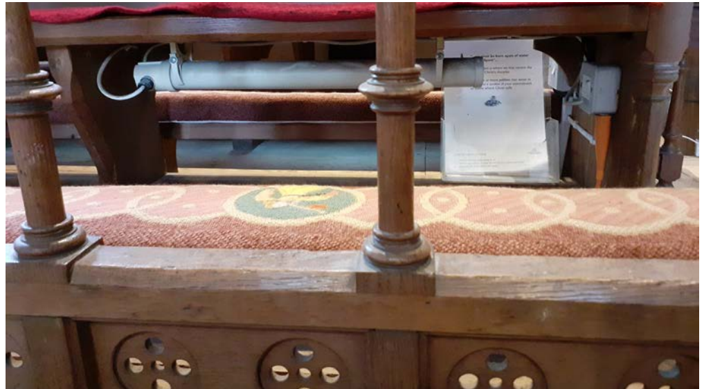
Figure 90: Radiant tube pew heater.
