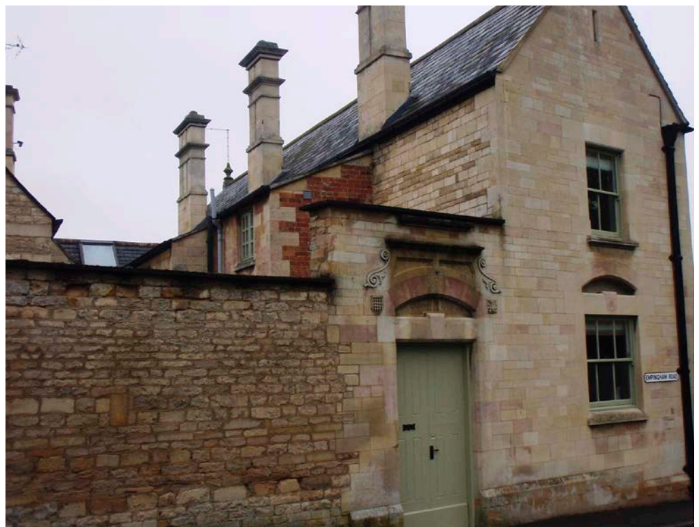
Figure 7: Hibbins House, Ketton. Ketton Stone.
