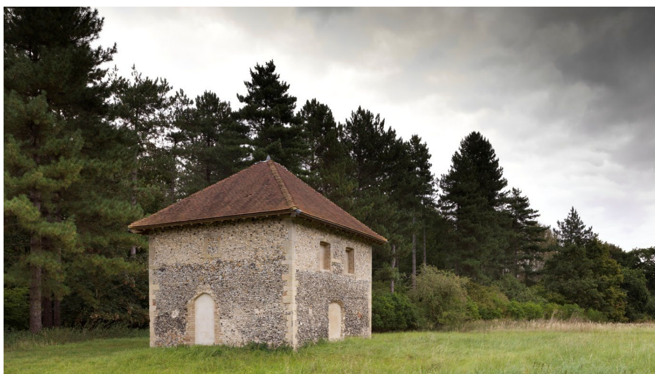
Figure 21 (above): Forestry England have recently completed works to this early fifteenth-century tower house in Mildenhall Forest, part of Thetford Forest in East Anglia. The house was originally used by the Warrener (the grounds keeper responsible for breeding and managing rabbits). The recent repairs have secured its condition, and research by the Breckland Society and Friends of Thetford Forest has helped to develop our understanding of the ancient use of the land and its agricultural past. The Mildenhall Forest Plan for 2024-34 allows for active monitoring of the landscape and the structures within it. [© Forestry England]
