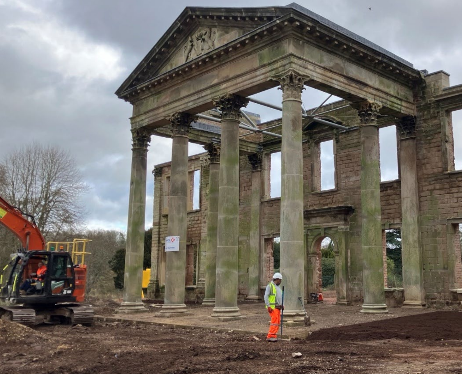
Figure 14 (above): Extensive repair and stabilising work to the ruins of Old Hewell Grange in Worcestershire, carried out over many years, was concluded in 2025-26. The building, originally built in 1712 by Francis Smith of Warwick with a portico by Thomas Cundy added in 1815-16, was reduced to a ruin in 1889 after fire damage caused by a fireworks display. The three remaining outer walls survive in Hewell Grange Park, to which the ruins of Old Hewell Grange make a significant contribution. [© Bromsgrove District Council / Mary Worsfold]
