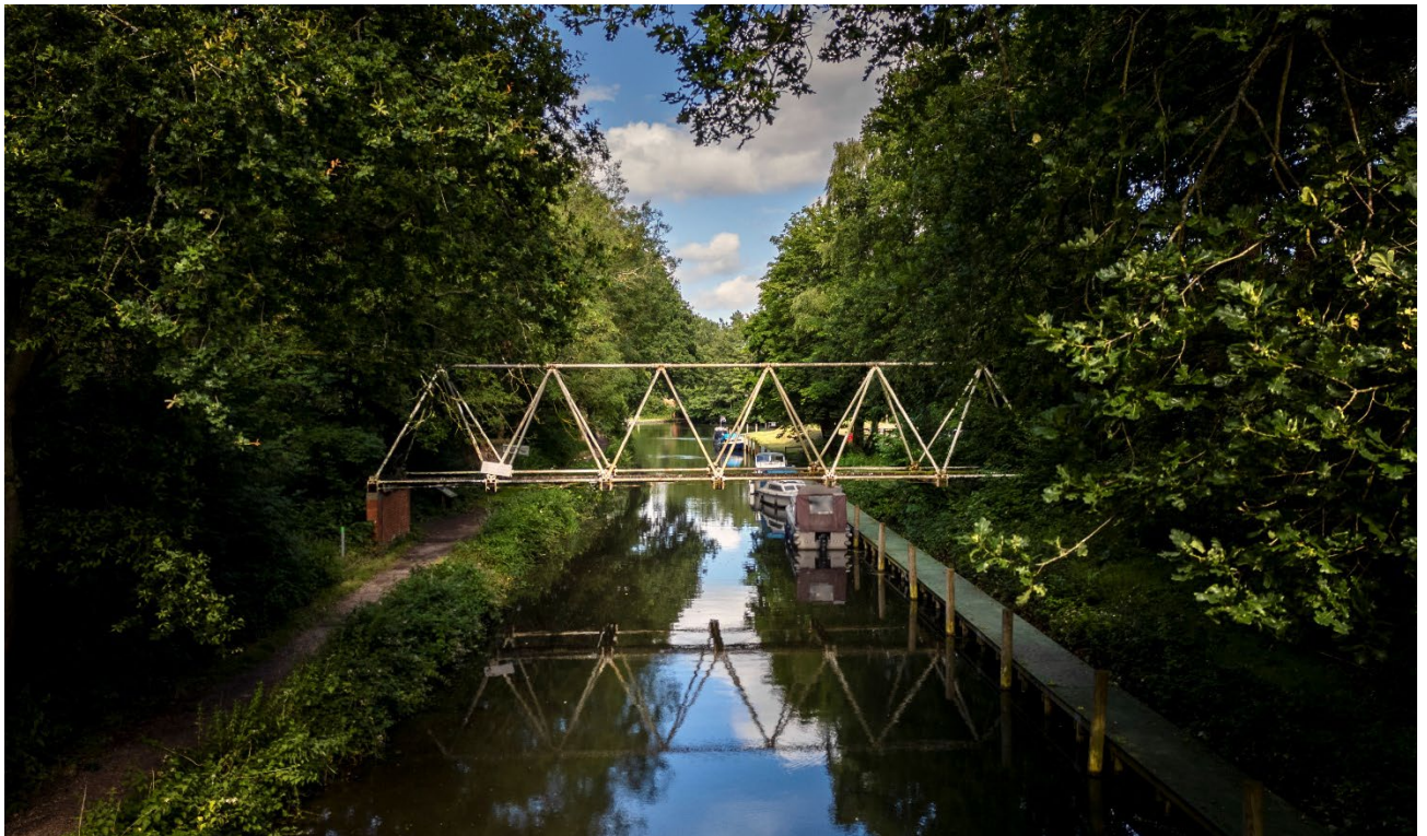
Figure 4: Crossing the Basingstoke Canal, the Inglis Portable Military Bridge (Light Type), is a rare survival of military structures in England that date from the First World War. Made of lightweight steel, it was quick and easy to construct with little training and could be reused, making it particularly appealing for use by the military. The design was still used in the Second World War and hugely influential in developing future military bridges. This original example, thought to have been brought back to Aldershot from France, was listed at Grade II in 2024. [© Historic England / Chris Redgrave]
