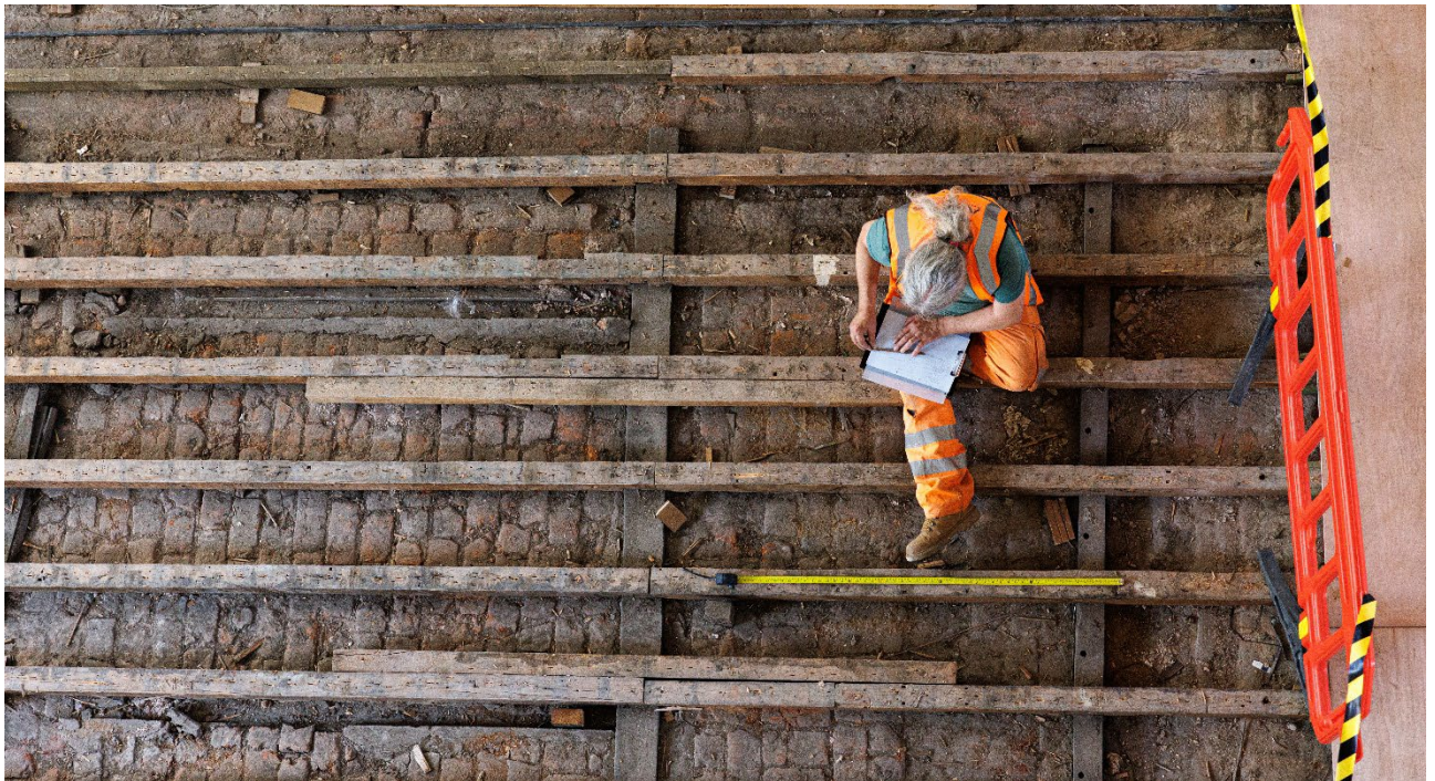
Figure 13: The recent conservation project at the Banqueting House in Whitehall (see Figure 12 on p.22) enabled careful recording of the original floor structure and the 1960s interventions before re-boarding with wide English oak boards. [© Historic Royal Palaces]
