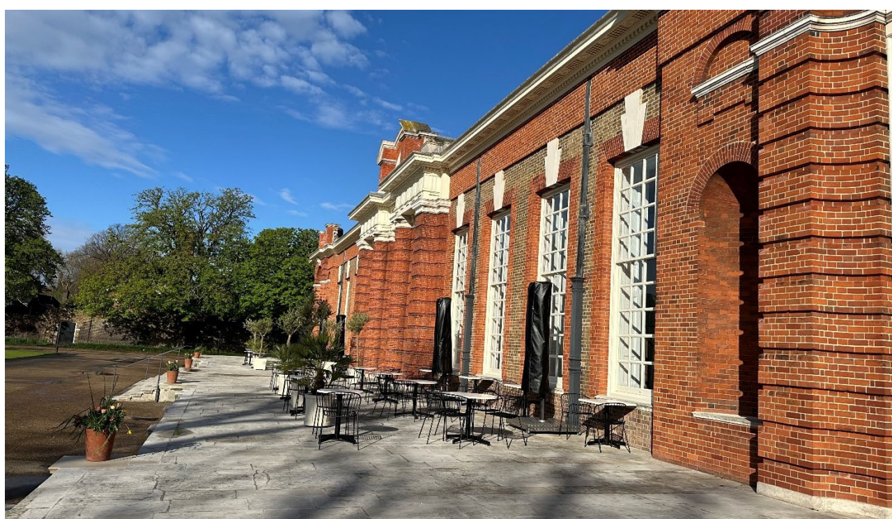
Figure 28: The Kensington Palace Orangery in London reopened in 2024 with terrace repairs forming the final phase of an extensive building project to repair the building and bring it back into use as a restaurant. The stone was repaired, repointed and cleaned with some limited replacement before works to the ramp's iron rails and new handrails to the central steps were fitted. [© Historic Royal Palaces]
