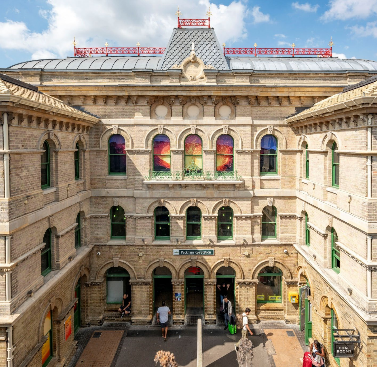
Figure 9: The restoration of the exterior of the Grade II listed Victorian station at Peckham Rye in London was the subject of considerable investment from Network Rail, the Railway Heritage Trust and Southwark Council. Working carefully from historic plans and photographs, as well as surviving historic fabric, the original roof materials and design were reintroduced and the elevations cleaned and repaired. The restoration project won a National Railway Heritage Award and ‘Best heritage roof’ award in 2023. [© Network Rail]
