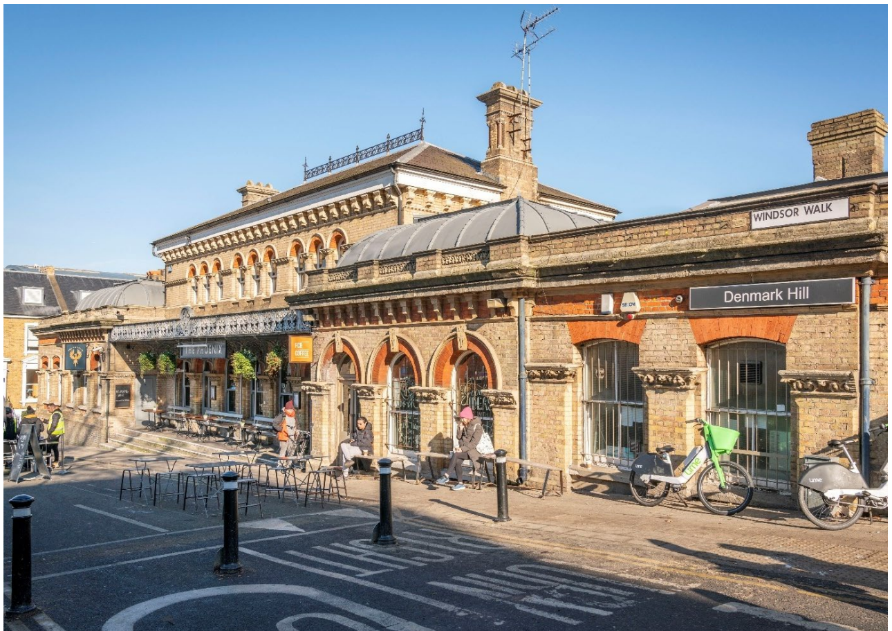
Figure 33: The Grade II listed Victorian station at Denmark Hill, London has been extensively repaired, with a new entrance on Windsor Walk supported by The Railway Heritage Trust. Works included the rebuilding of the listed wall to its original design and gates, and the introduction of a photovoltaic film to the roof to generate renewable energy. The station was removed from the national Heritage at Risk Register in 2024. [© Network Rail]
