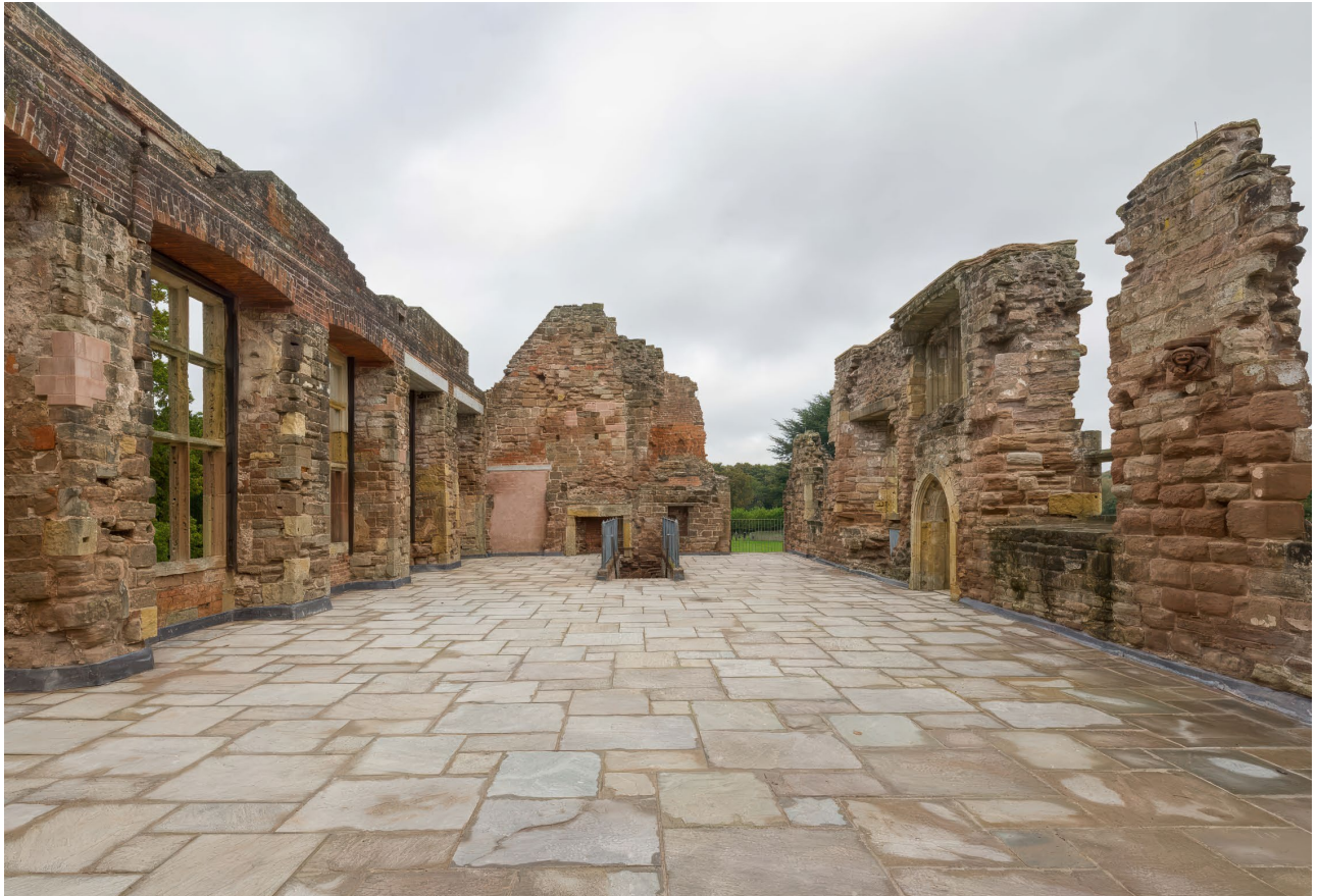
Figure 11: A programme of repairs to the west range of Rufford Abbey in Nottinghamshire has enabled it to re-open to the public. Works included a new waterproofing solution to prevent further moisture ingress to the twelfth-century Fraternity Undercroft. The remains are among the best preserved in the country and form part of Rufford Abbey Country Park, a popular tourist attraction. [© English Heritage Trust]
