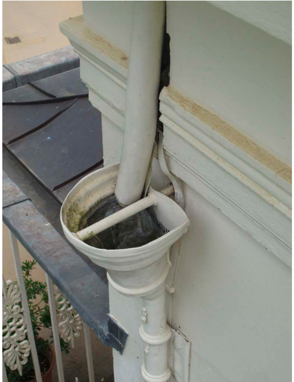
Figure 53: Hopper head and rainwater pipe from parapet gutter on north side of building.
