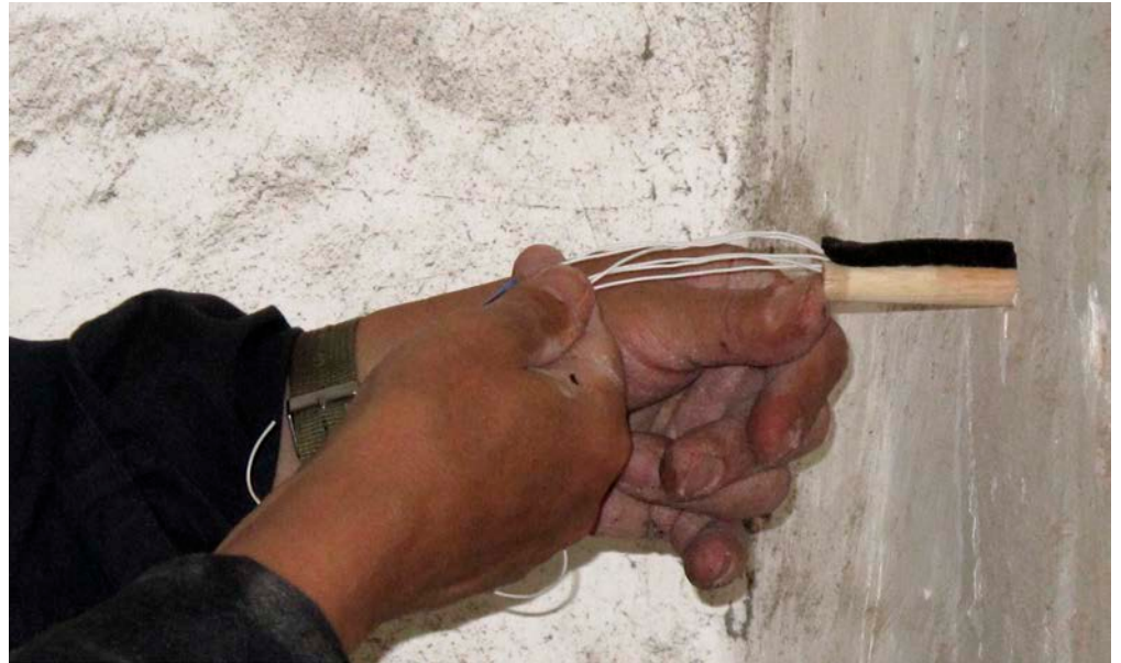
Figure 28: Inserting segmented timber dowel into a hole drilled in wall.
