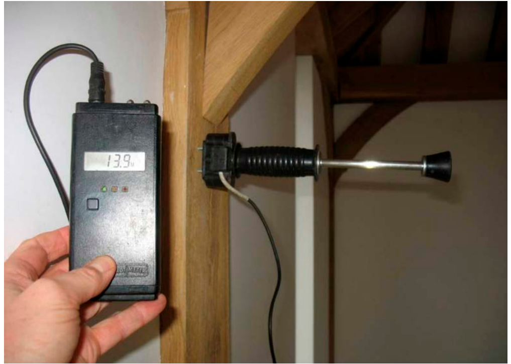
Figure 36: A hammer probe has electrodes that are insulated, except at the tip. These can be driven into the timber to various depths to provide a moisture gradient.
