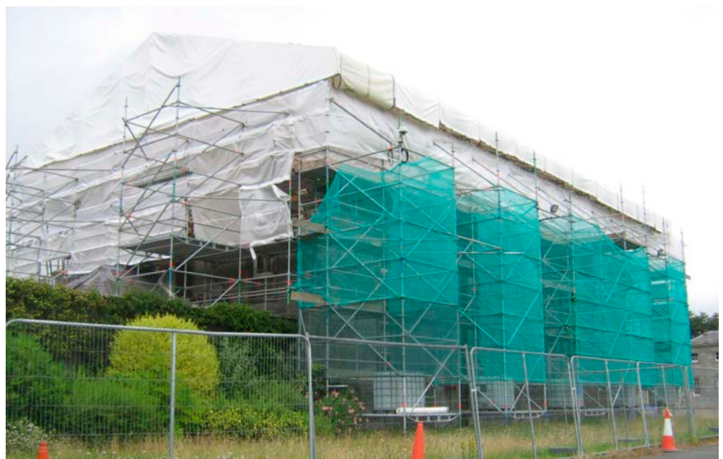
Figure 44: Temporary roof and weatherproofing designed to maximise ventilation.
