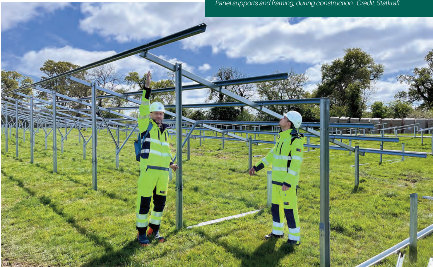
Panel supports and framing, during construction . Credit: Statkraft
