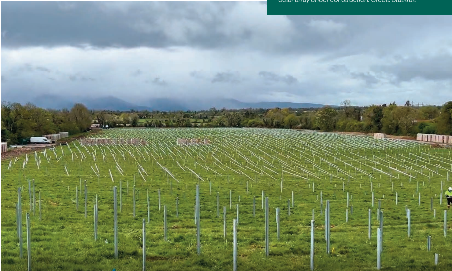
Solar array under construction. Credit: Statkraft
