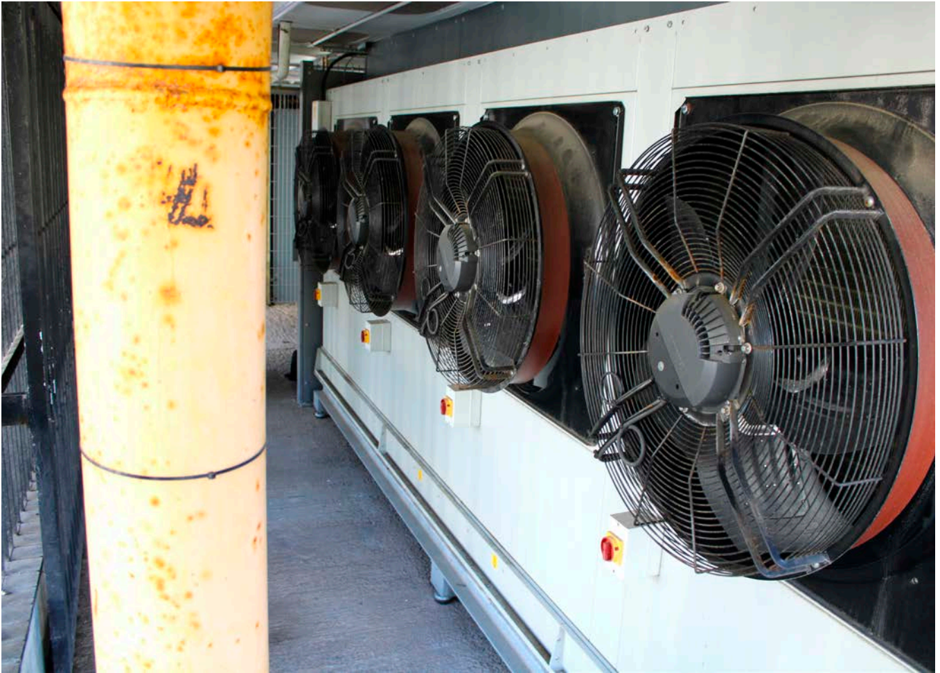
Figure 18: One of four sets of ASHP evaporators (right), pictured with the gas main (left).
