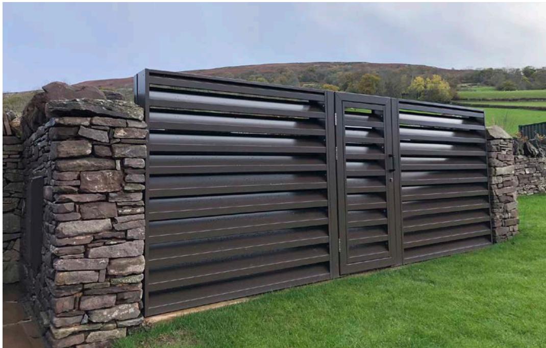
Figure 13: ASHP enclosure at Site 2.
