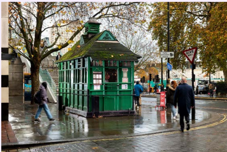
Cabmen's Shelter, Northumberland Avenue at the junction with Embankment Place, London. Grade II listed
