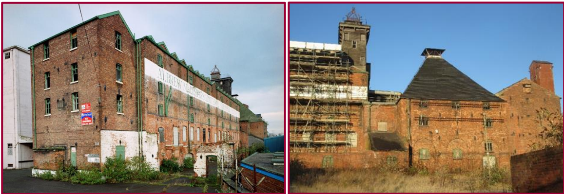
Figure 2-2 Site conditions prior to Heritage Fund investment
