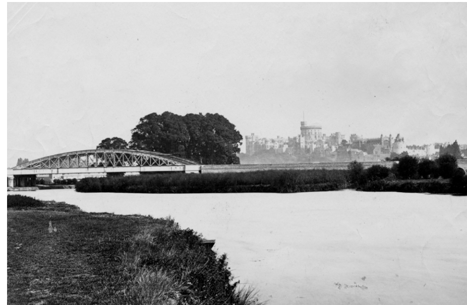
Fig. 57: One of the railway bridges carrying the Great Western Railway over the river Thames, with the buildings of the Castle in the distance, 1870 [Source: Historic England Archive]
