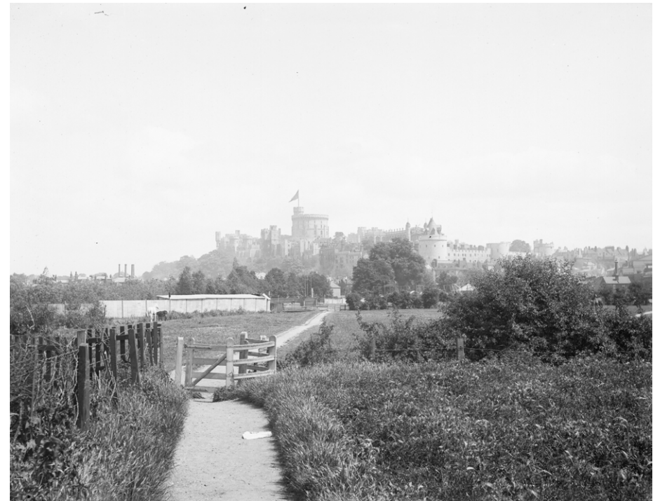
Fig. 30: The undeveloped Clewer Meadows in the late-nineteenth century [Source: Historic England Archive]
