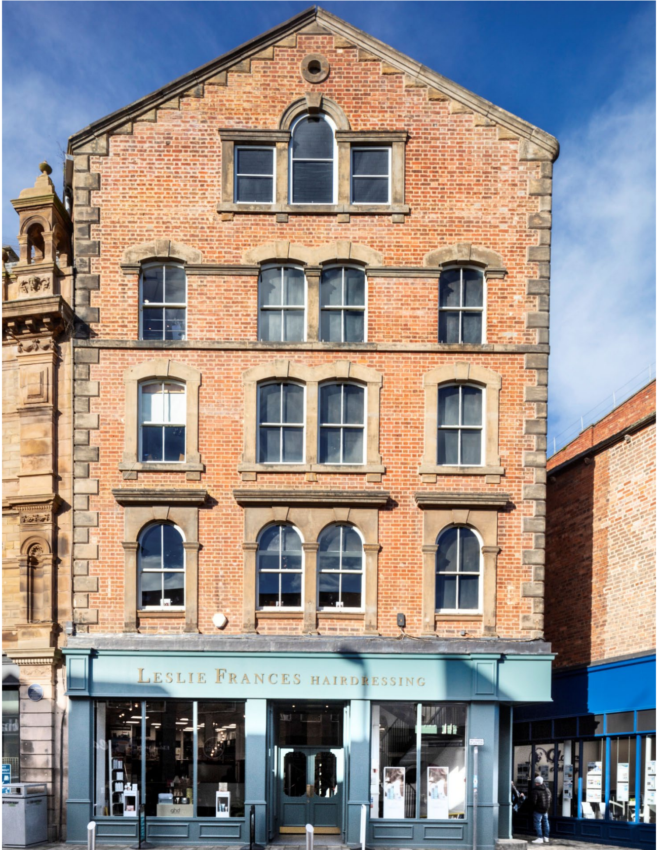
258 Eldon Street, Barnsley, South Yorkshire. Included on the South Yorkshire Local Heritage List. Alan Bull © Historic England Archive DP486478
