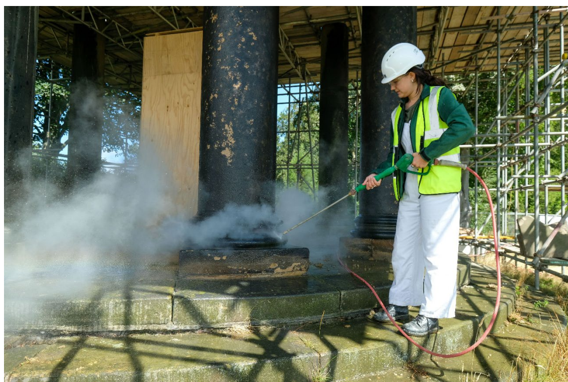
Figure 9: A trainee working on the Ionic Temple at Wentworth Woodhouse, during the 2022 HBS Summer School, ©Historic England
