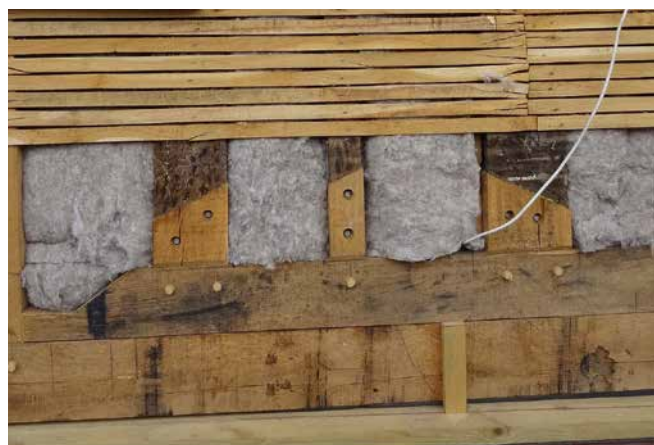
Insulation in a timber-framed wall.
