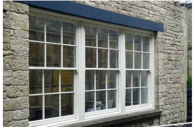
Timber sash windows, The Engine House, Swindon.
