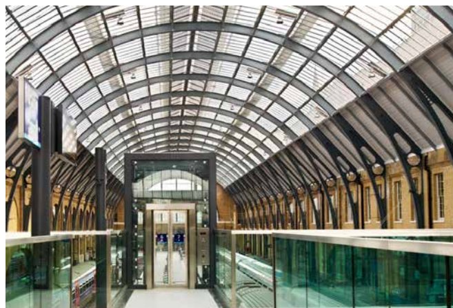
Photovoltaic cells installed in the glass roof above King's Cross Station, London.
