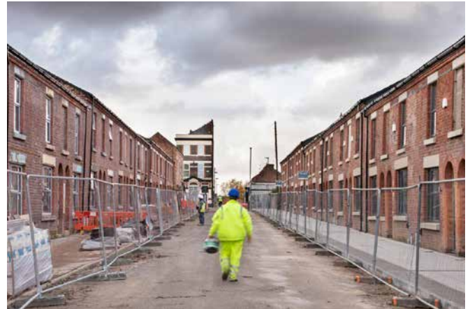
Regeneration of Victorian terraced housing in Toxteth, Liverpool.
