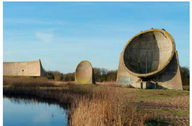
Concrete sound mirrors near Dungeness, Kent.
