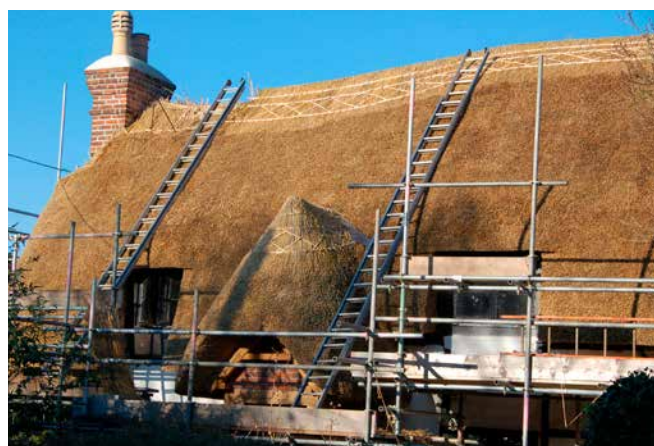
Re-thatching a cottage.
