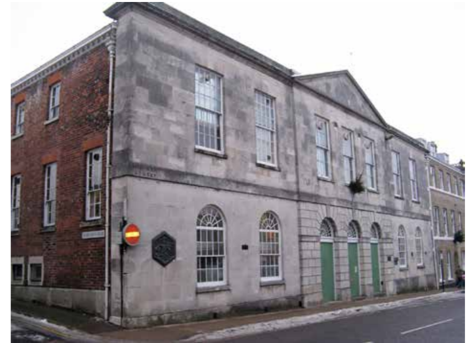
Shire Hall before the 2018 refurbishment works Image source: Philip Hughes Associates
