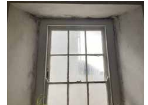
Mould around flat window
