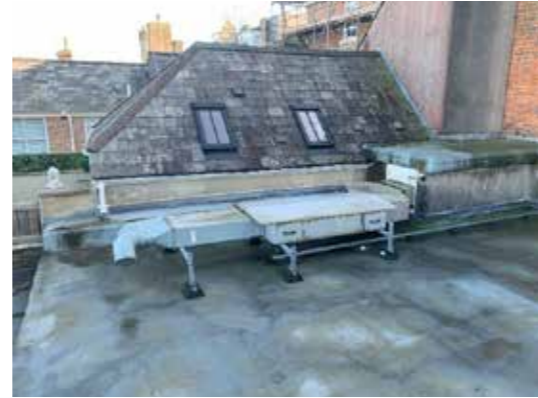
Left: MVHR unit located on low rear roof assumed to serve basement museum areas. Access up to unit not possible. Right: assumed system controller location in store at basement level.
