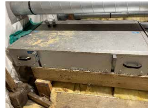
MVHR unit in roof void assumed to serve grand Jury room
