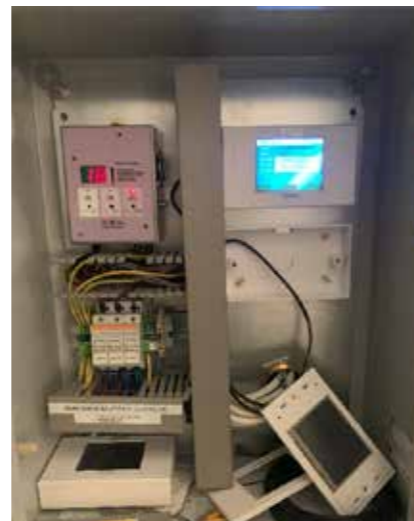
Grand Jury Room fan controller disassembled
