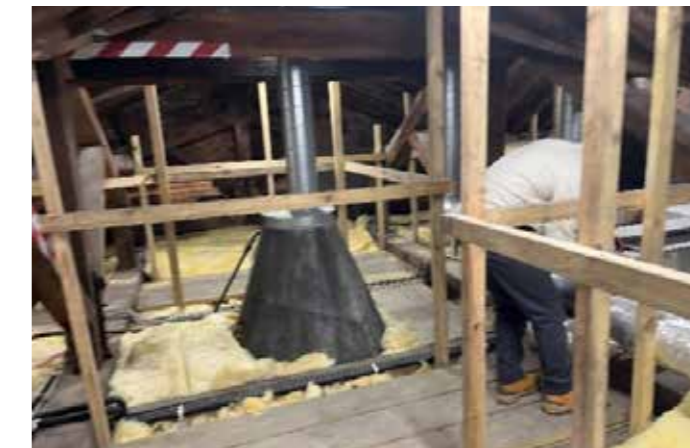
Ductwork connection onto ceiling grille in roof void.
