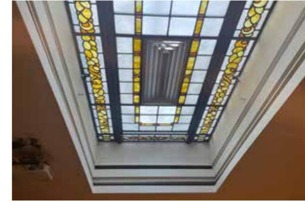
Open ventilation grille in centre of rooflight to learning space. Glazed lantern at roof level above rooflight.
