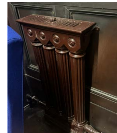
Ornate radiator in Silence Room
