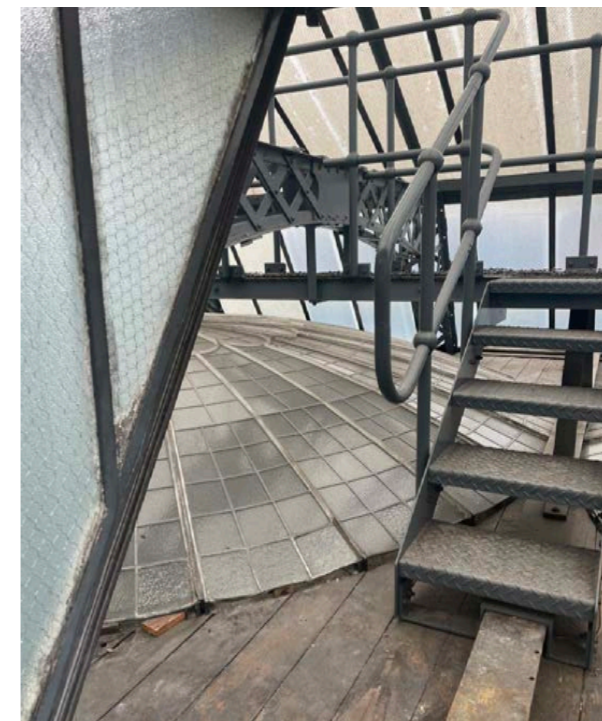
Single-glazed roof lanterns over decorative laylights
