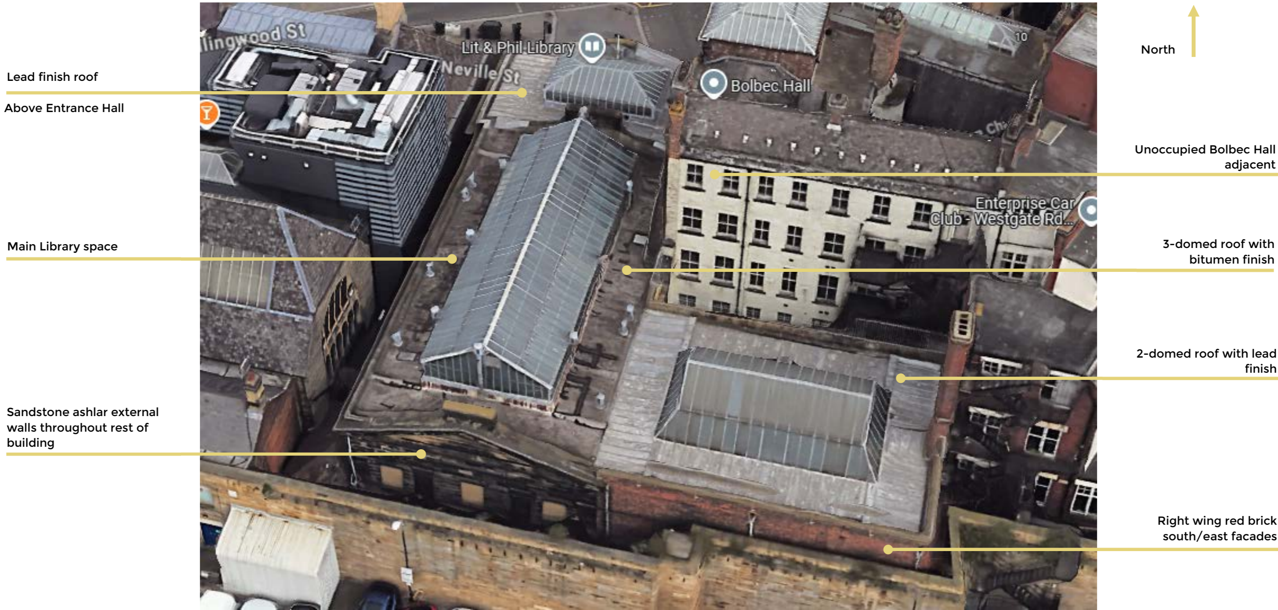
Satellite view of Lit & Phil Library with key zones indicated and external fabric Image Source: Google Earth
