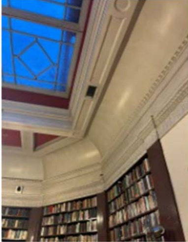
Ventilation air ducts integral to beams
