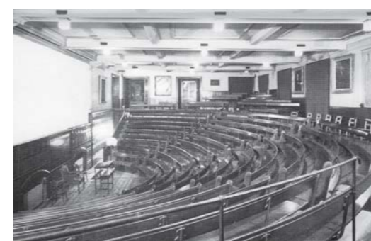
The lecture theatre 1866-1967, shortly before its removal
