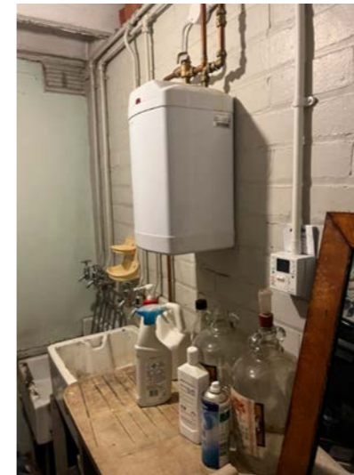
Local electric water heater visible in basement store
