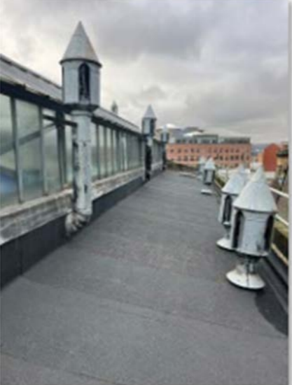
Air ducts integral to Library ornate plaster ceiling (left) connected to Victorian turrets on roof (right)
