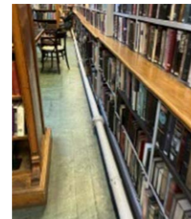
Exposed pipe throughout library space
