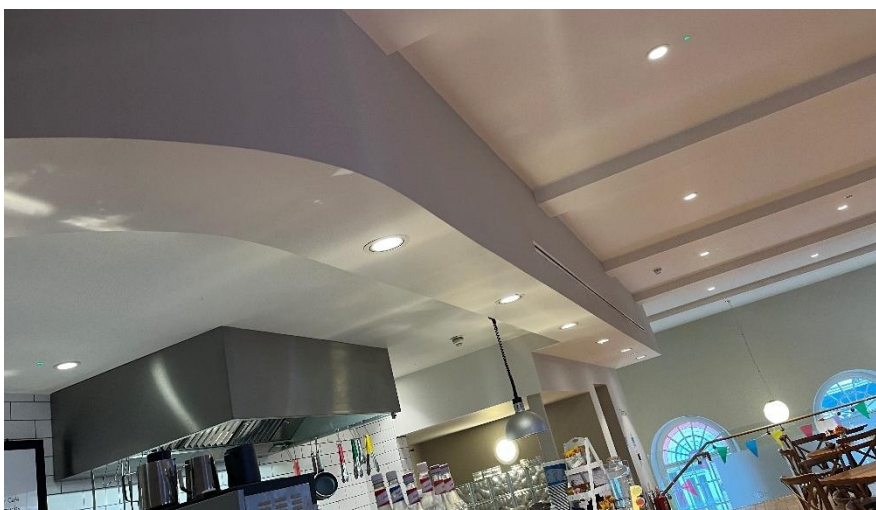
Figure 5-13 - Cafe supply & extract ventilation
