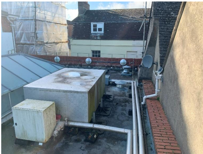
Figure 5-3 Possible water tank on Learning space roof. Access not possible.
