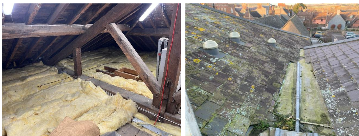
Figure 7-1 Left: Roof insulation. Right: Sun tubes penetrating pitched roof
